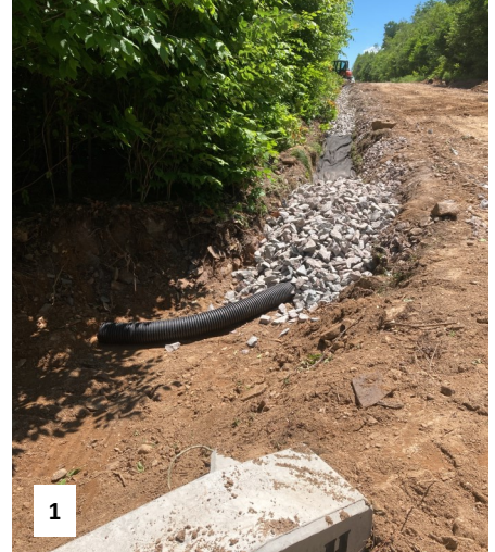
Photo 2 - Completed road section with multiple cross pipes
