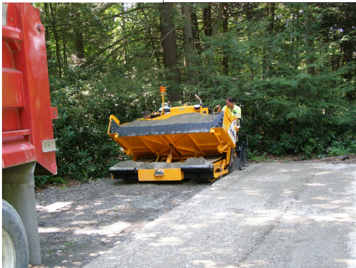
Installing driving surface aggregate with a paver in Polk Township.
